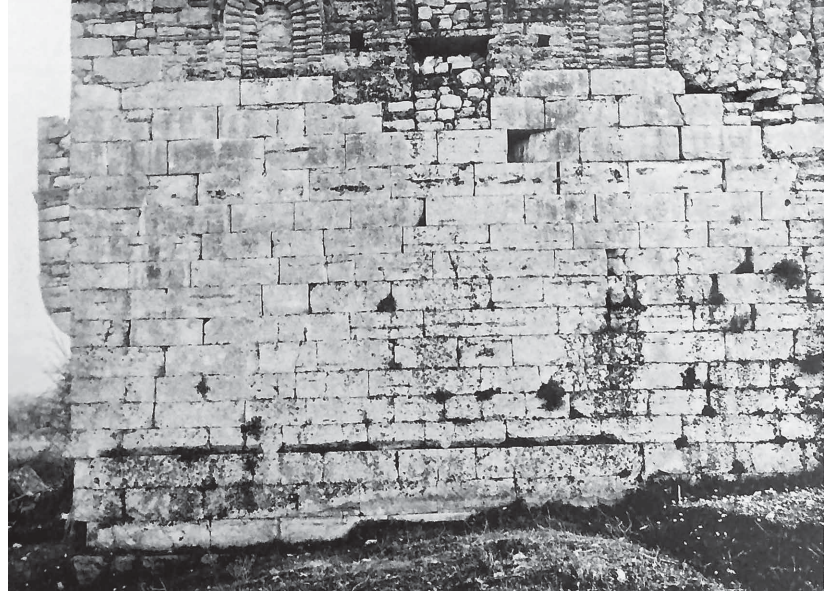
Figure 39. Isodomic ashlar masonry of the fortification tower and wall at the Church of Panayia Nerantzicha, Corfu (Korkyra). Korkyra 1, pl. 1; courtesy Verlag Gebr. Mann, Berlin
