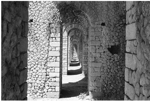
FIGURE 2.26 Detail of terrace substructure with arches enfilade, Terracina; Photo: antonioa89 via Wikimedia.
