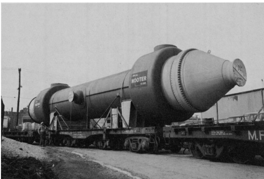
Photograph 1.k. Heat exchanger with enlarged shells at nozzle entry and exit. (Courtesy Nooter Corporation, St. Louis, Missouri.)
