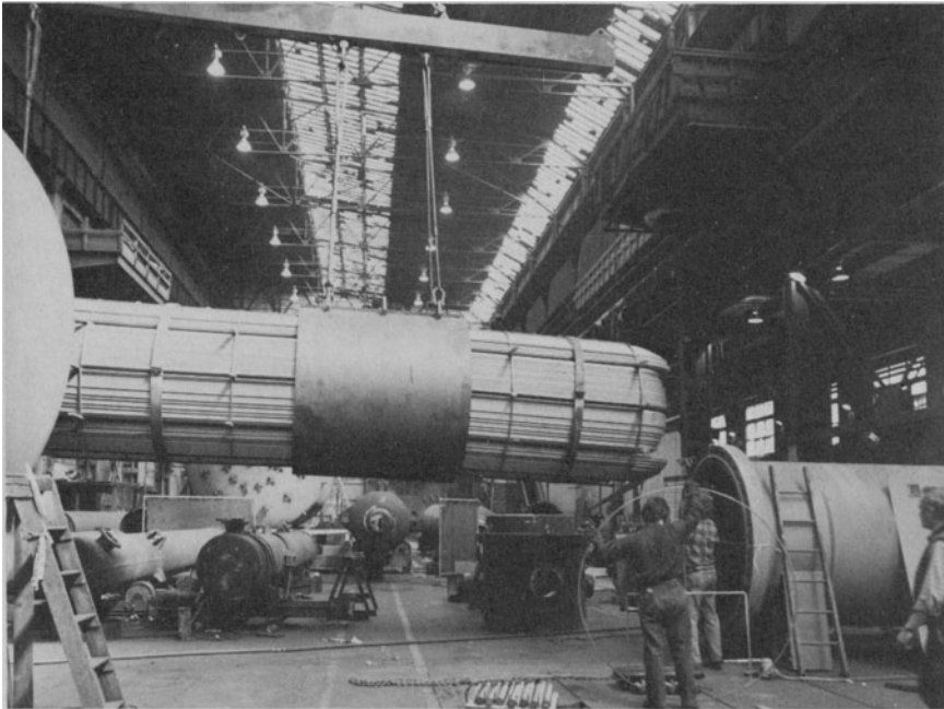
Photograph 22.d U-tube bundle being lifted with special “belly band” rig. (Courtesy Joseph Oat Corporation, Camden, NJ)
