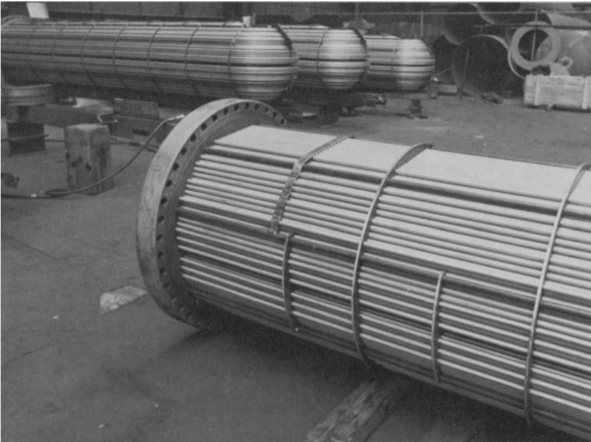
Photograph 16-d. Field fix of tube span in front of shell inlet.
