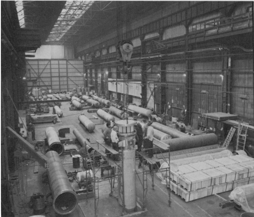
Photograph 22.c. Vertical bundle insertion. (Courtesy Joseph Oat Corporation, Camden, NJ)
